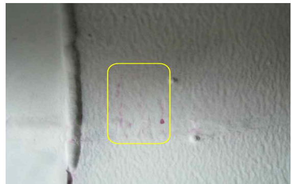
Fig. 5 Using the penetration test pipe internal defect detection
