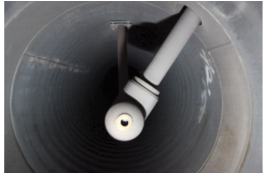
Fig. 5 Imaging Probe Installed in the Diffuser
