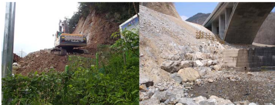
Fig. 12. Cutting trees during construction.
