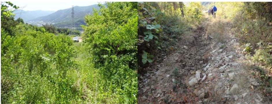
Fig. 9. Weeds overgrowth (left) and soil erosion (right) on the access/management road.
