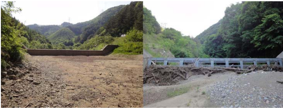
Fig. 13. Sediment and in-stream wood stored by the check dam.
