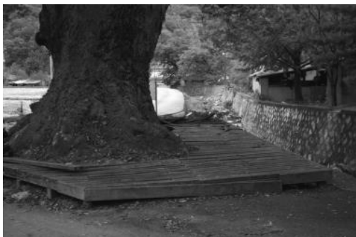
a. Existing condition before construction
