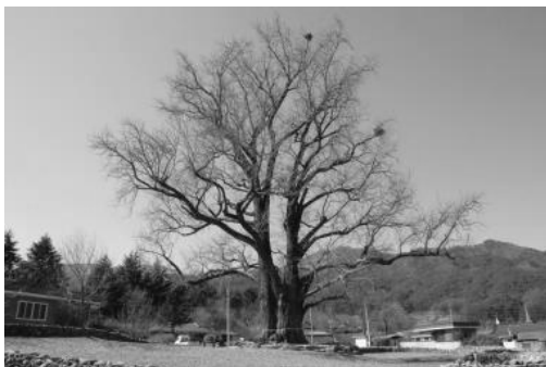
a. Existing condition before construction
