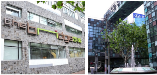
Fig. 3. The Factory Remodeling in The bridge 8
