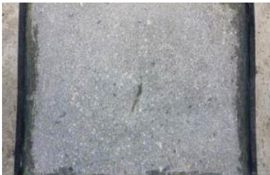
Fig. 15. Surface condition after finishing test
