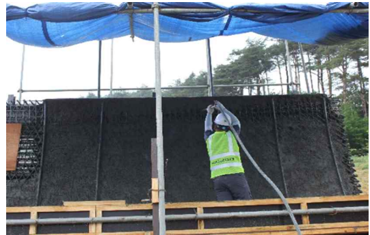
Fig. 6. Rebound elimination using air
