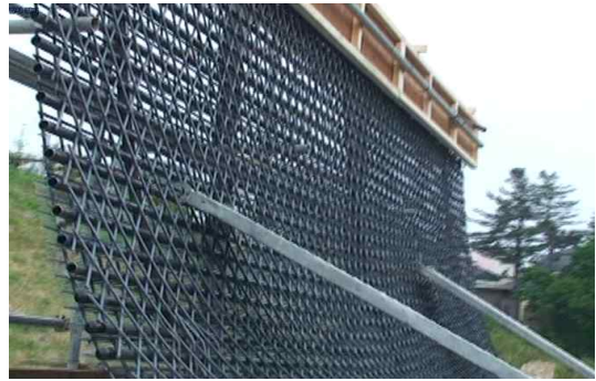
Fig. 2. Foreground of Installed Rebar
