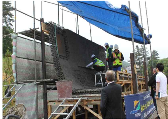
Fig. 10. Screed finishing
