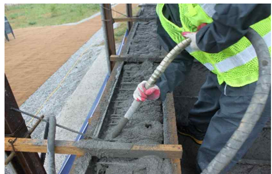
Fig. 7. Vibrofloatation using vibrator
