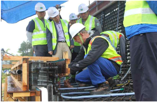
Fig. 4. Reinforced state checking
