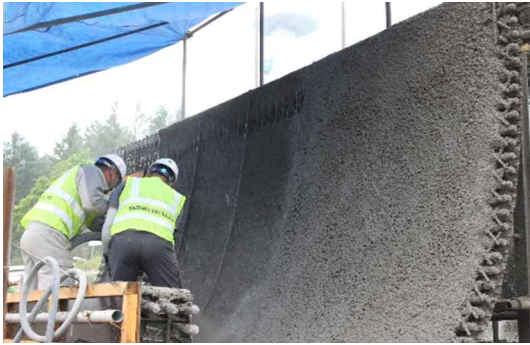
Fig. 8. Placing a secondary surface shotcrete
