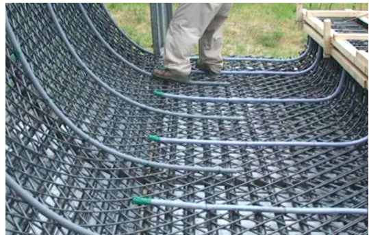
Fig. 3. Foreground of Installed Standard Pipe
