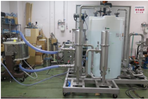
Fig. 11. The system for removal of iron oxide scale from feed water in thermal power plant using magnetic separation.
