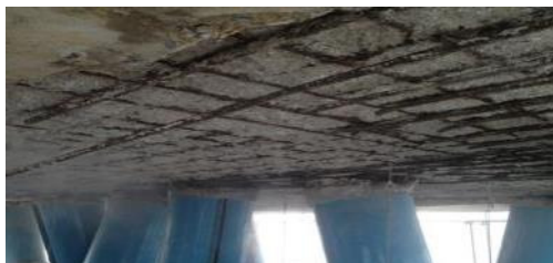
Fig. 2. The Illustration of Harbor Structures Concrete Deterioration [1]
