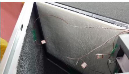
Fig. 11. A photo of freezing in case of -20^{\circ}\text{C} of OA temperature and 22^{\circ} open of recirculation damper.
