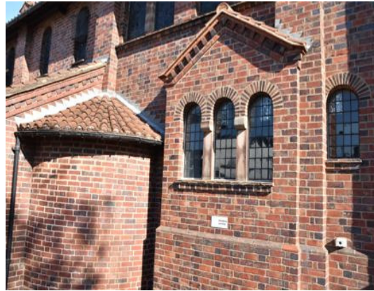
Fig. 8. St. Andrews Church Detail (Photo, 2018)
